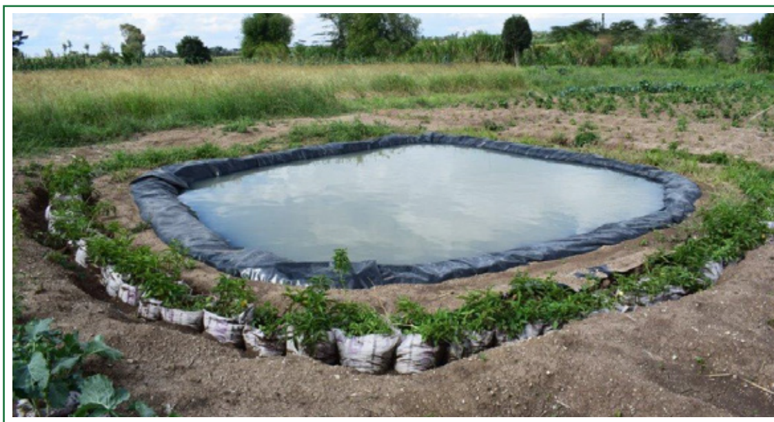
Figure 3: A lined water pan; it took this group 8 hours to excavate the pan
